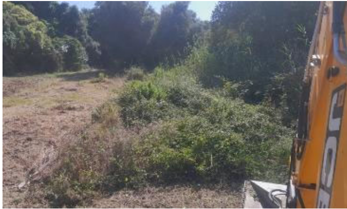
Example of vegetation clearance works using a backhoe loader and a brush cutter
